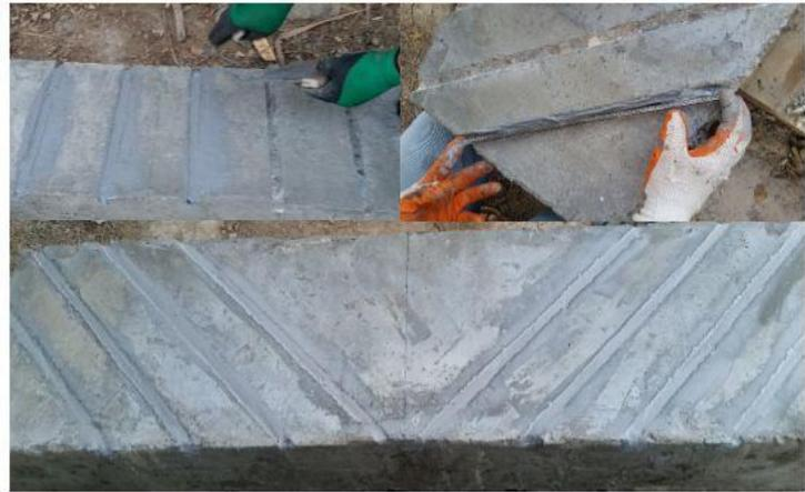
Figure (4) Imbedded Bars into Grooves
