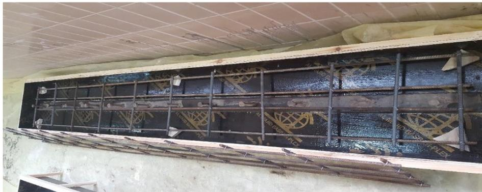
**Fig.2 Steel Reinforcement of Concrete Slab of Composite Beam**
