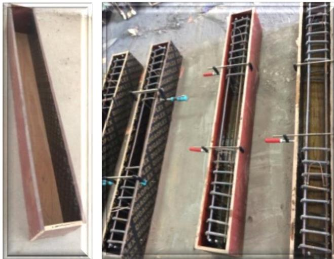
**Figure 1** Beam molds and reinforcement.
