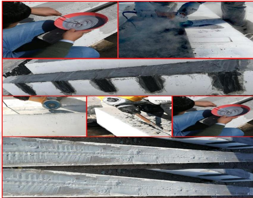
Fig. 3: Steps of applying BFRP sheets and NSM-GFRP bar.
