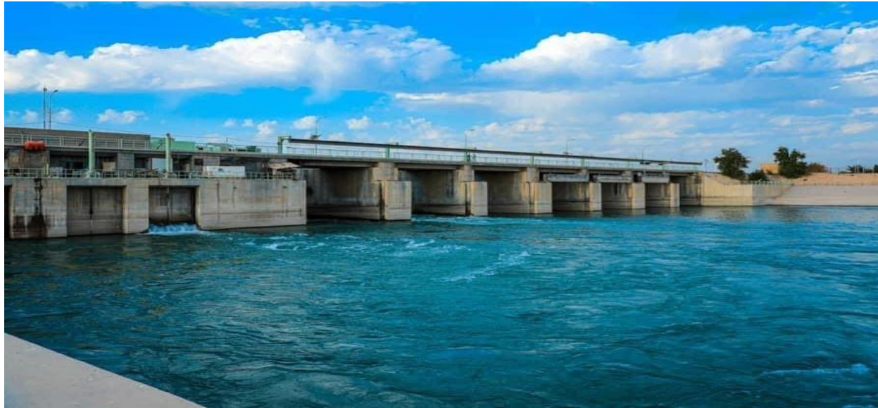
Figure (2) kufa barrage
