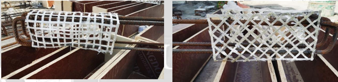
Fig. 2: Applying GFRP grid reinforcements to the steel cage
